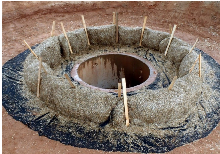
Figure IP-6 Wattle Inlet Protection Installation.
