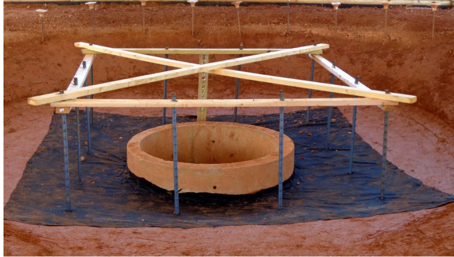
Figure IP-1 Silt Fence Inlet Protection Installation. (Showing geotextile underlayment, steel T-posts, 2 x 4 bracing, and dewatering device.) (Photo courtesy of AU-SRF. See Appendix for CAD files)
