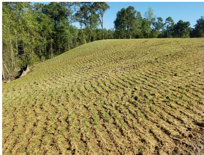
Figure LG-1 Tracked and Hydroseeded Slope
