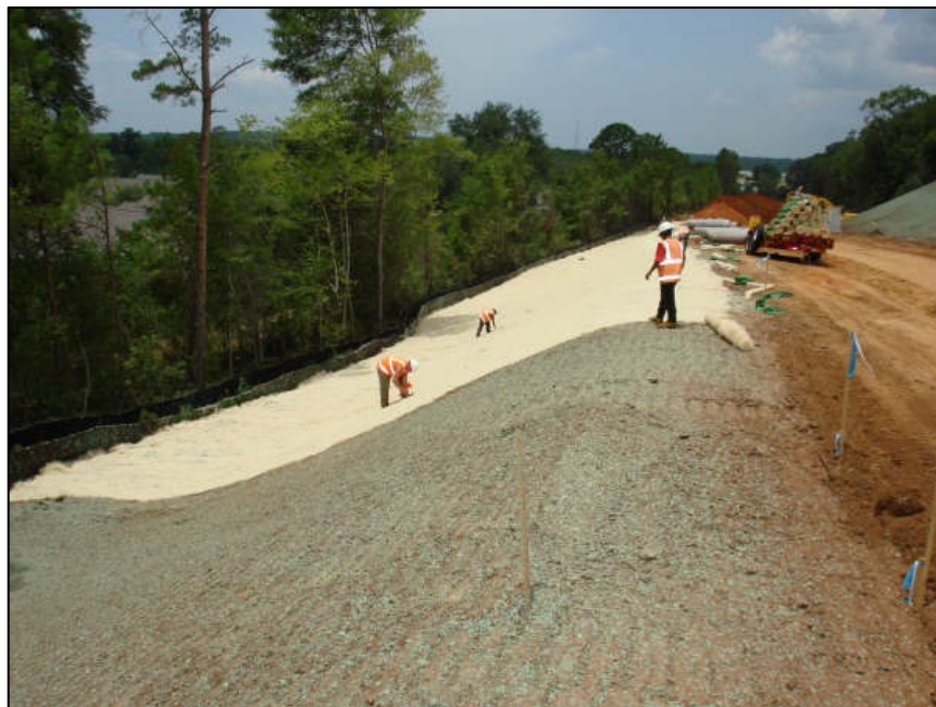
Figure ECB-1 RECP Slope Installation. Photo courtesy of John Slupecki.
