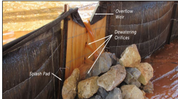
Figure SB-3 Example dewatering board & overflow weir.
