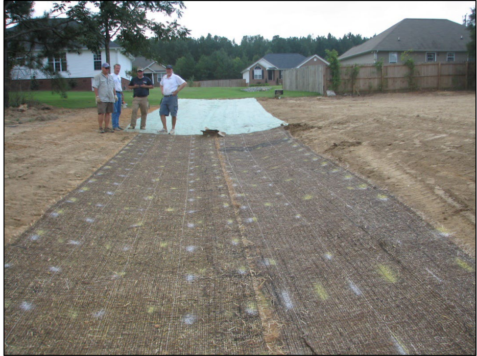
Figure ECB-4 TRM with Pre-Marked Stapling Pattern.
