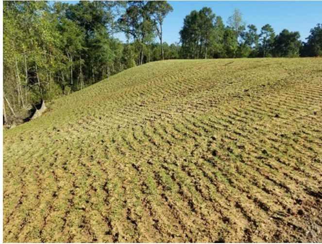
Figure LG-1 Tracked and Hydroseeded Slope
