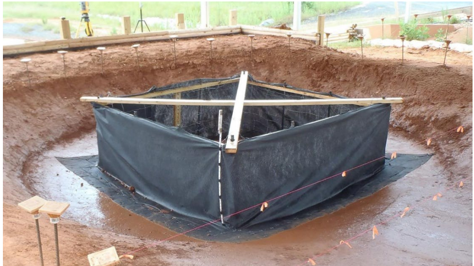
Figure IP-1 Silt Fence Inlet Protection Installation. (Showing silt fence, geotextile underlayment, steel T-posts, 2 x 4 bracing, and dewatering device.)
