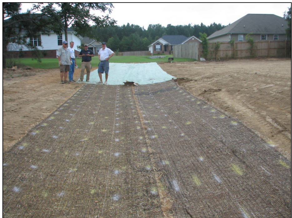
Figure ECB-4 TRM with Pre-Marked Stapling Pattern.
