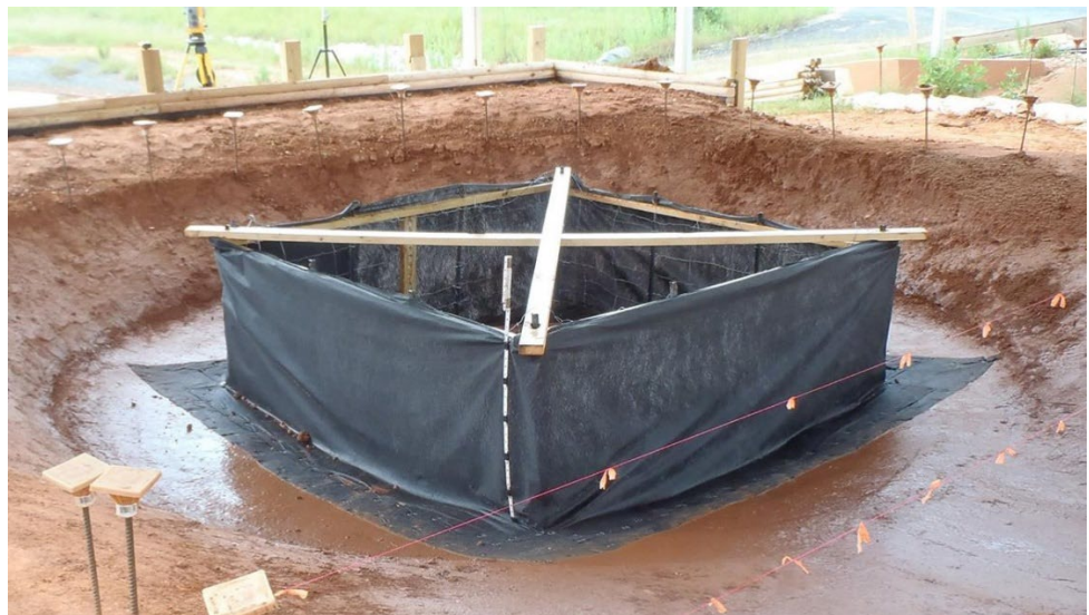
Figure IP-2 Silt Fence Inlet Protection Installation. (Showing silt fence, geotextile underlayment, steel T-posts, 2 x 4 bracing, and dewatering device.) (Photo courtesy of AU-SRF. See Appendix for CAD files)
