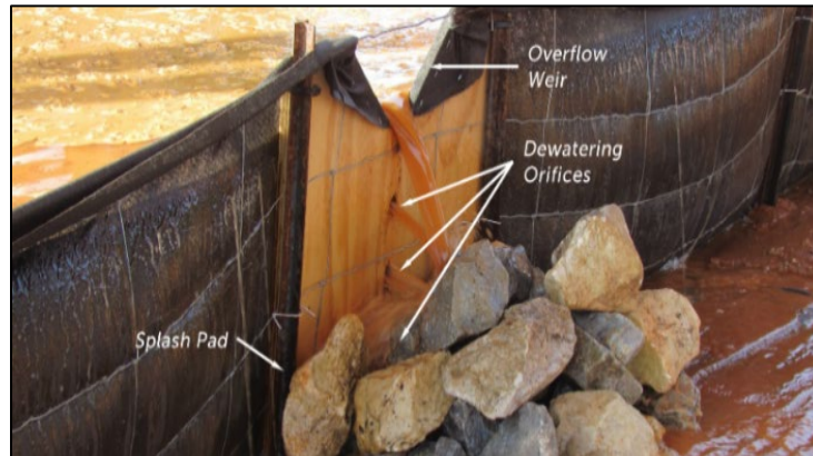
Figure SB-3 Example dewatering board & overflow weir.
