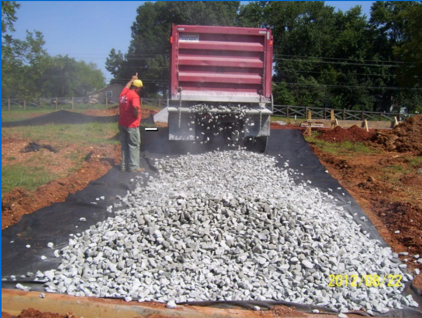
Construction Exit Pad
