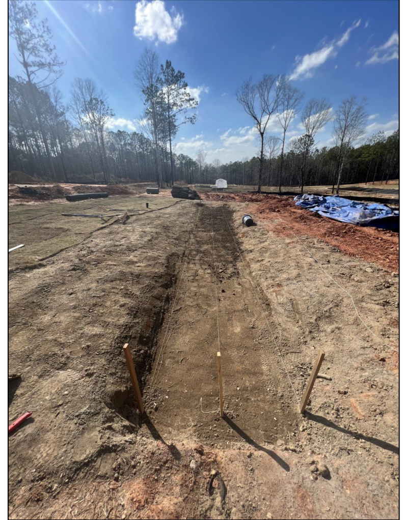
1% Grade & Channel Shaping
