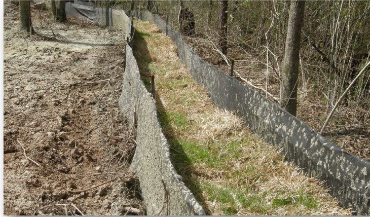
Sediment Retention Barrier
