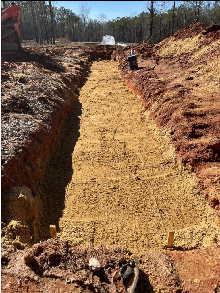
Fill 2 ft of Sand and Grade at 1% Slope
