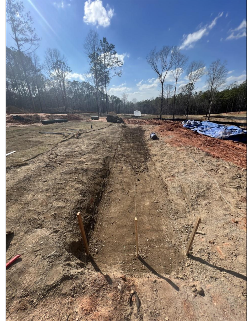
Grade Topsoil at 1% Slope
