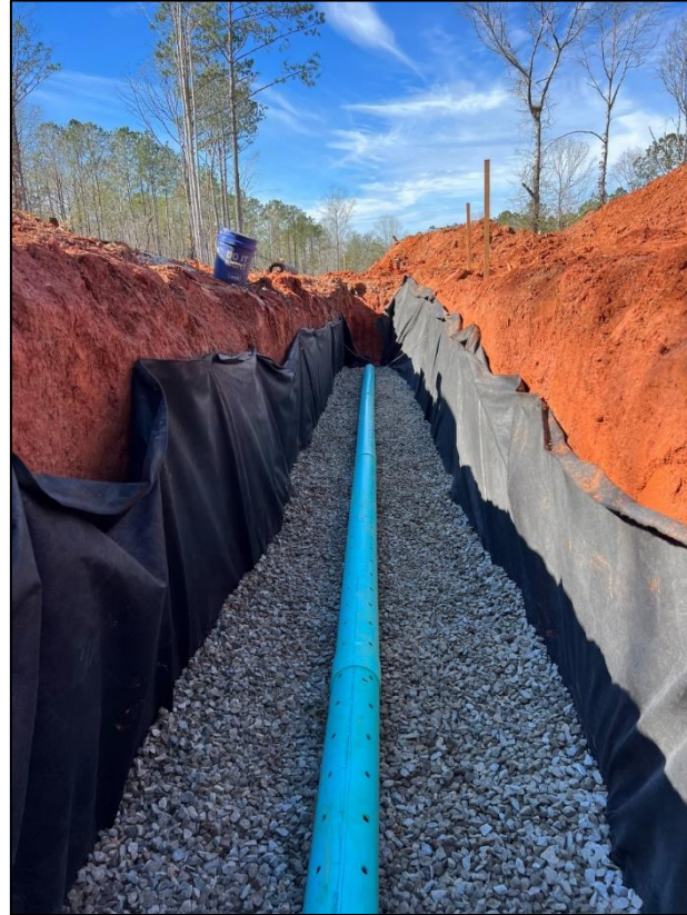
2 ft Fill of #57 and Underdrain
