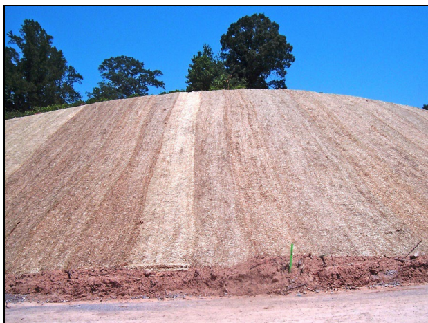
Figure ECB-1 Erosion Control Blanket on a Slope. Photo courtesy of Sunshine Supplies, Inc.
