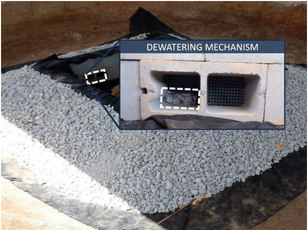
Figure IP-4 Block and Gravel Inlet Protection installation showing dewatering device.
