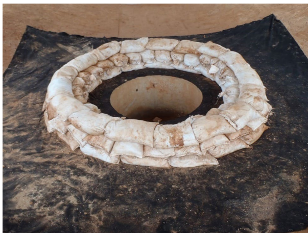
Figure IP-5 Sand Bag Inlet Protection installation. (Photo courtesy of AU-SWRF)
