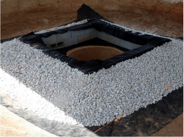
Figure IP-3 Block and Gravel Inlet Protection installation showing geotextile underlayment, gravel, and dewatering device.
