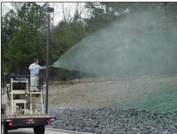
Figure CHS-1 Hydraulically Applied Flocculant.
