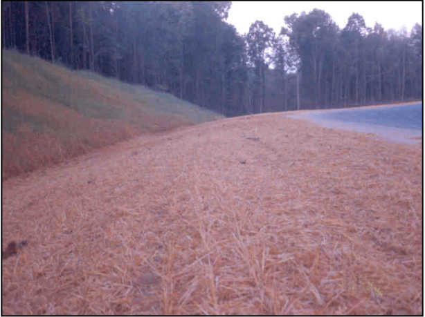
Figure MU-1 Crimped Straw Mulch.
