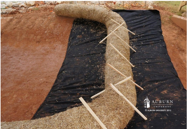
Figure CD-4 Wattle Check Dam
