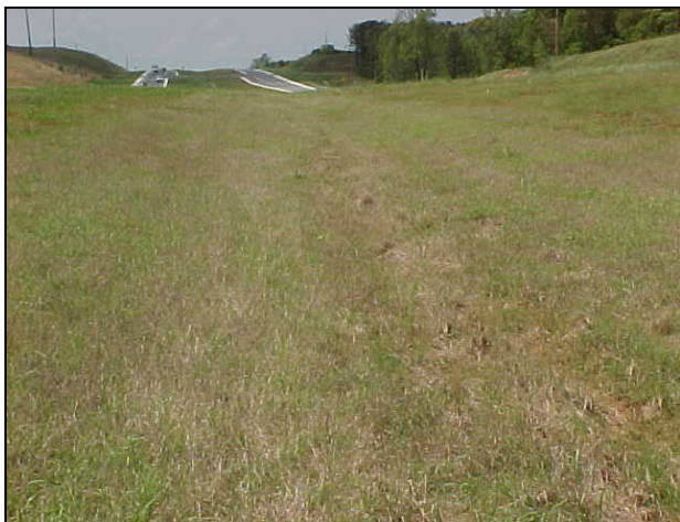
Figure GS-1 Grass Swale in a Highway Median.
