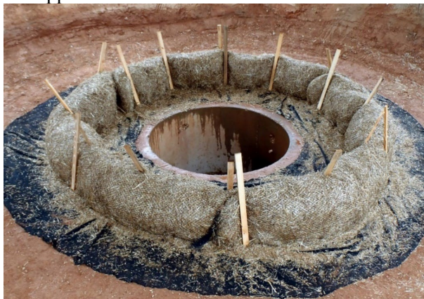
Figure IP-6 Wattle Inlet Protection installation. (Photo courtesy of AU-SWRF)
