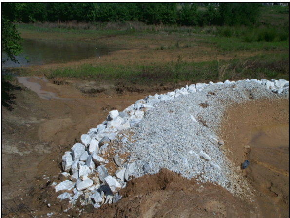
Figure RD-3 Typical Rock Filter Dam
