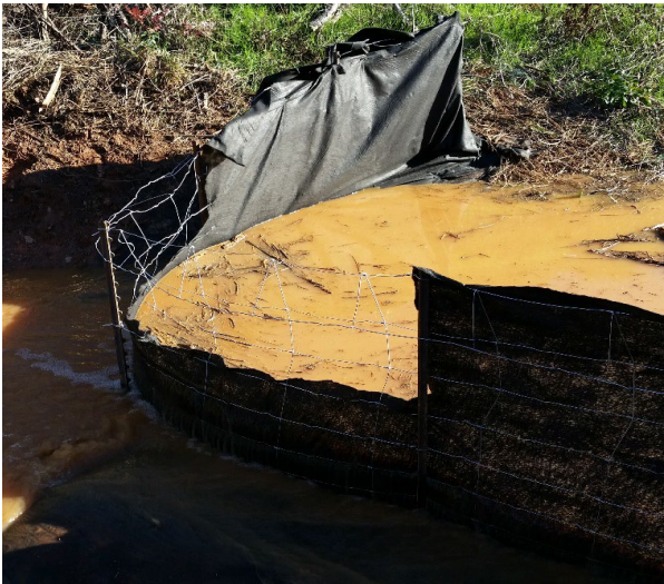
Figure CD-7 Silt Fence Check Dam
