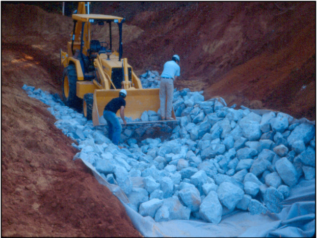
Figure RS-1 Hand Placing Riprap.
