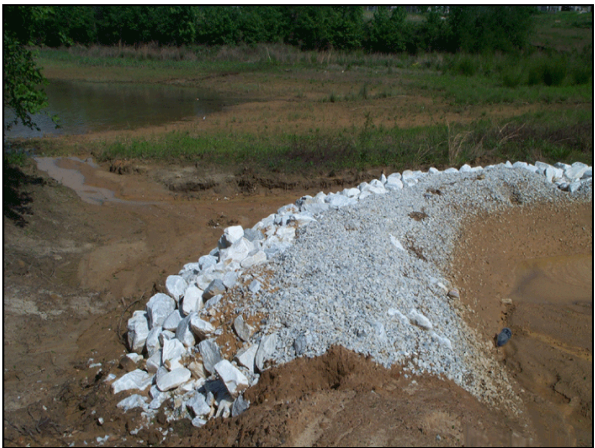
Figure RD-3 Typical Rock Filter Dam
