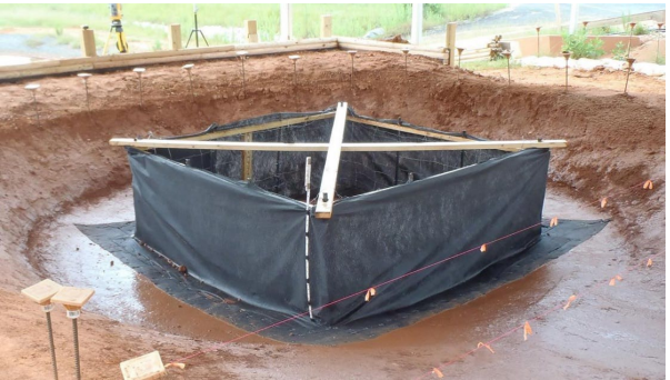
Figure IP-2 Silt Fence Inlet Protection installation showing silt fence, geotextile underlayment, steel T-posts, 2 x 4 bracing, and dewatering device.
