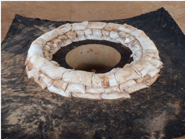
Figure IP-4 IP-5 Sand Bag Inlet Protection installation.
