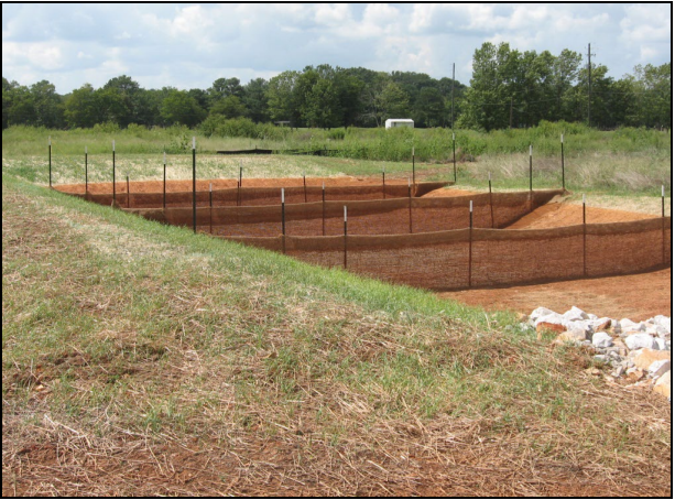
Figure SBN-3 Example of porous baffle made of 700 g/m 2 coir erosion blanket as viewed from the inlet
