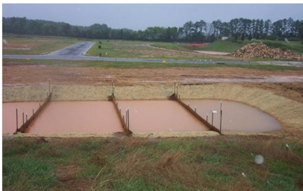
Figure EDS-1 Sediment Basin
