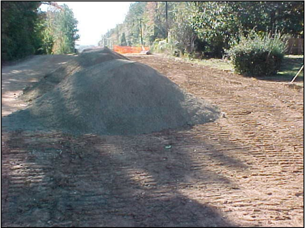
Figure TSG-1 Topsoil to be Spread.
