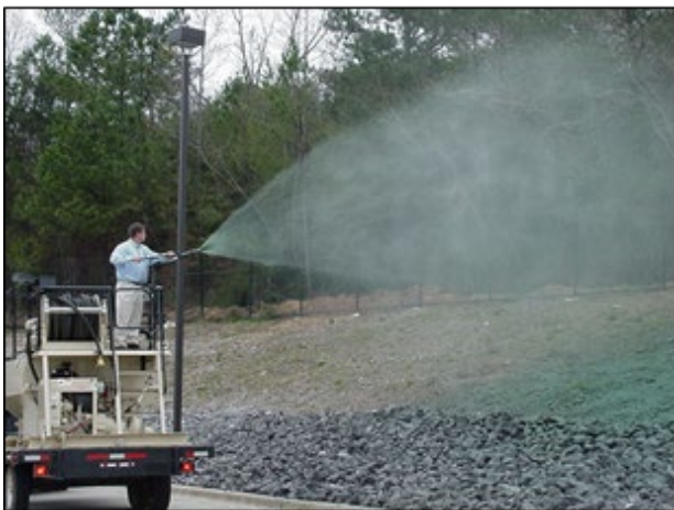
Figure CHS-1 Hydraulically Applied Flocculant.
