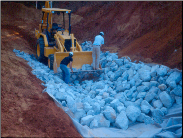
Figure RS-1 Hand Placing Riprap.
