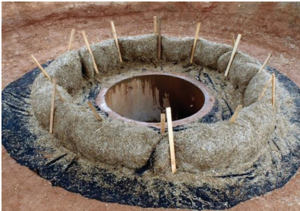
Figure IP-6 Wattle Inlet Protection installation. (Photo courtesy of AU-ESCTF)
