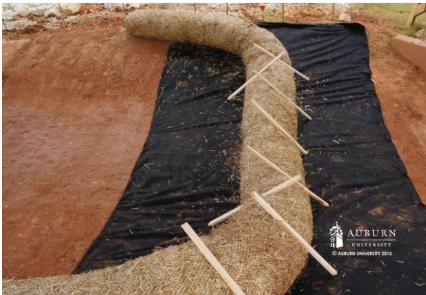
Figure CD-4 Wattle Check Dam
