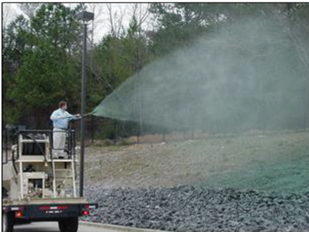
Figure CHS-1 Hydraulically Applied Flocculant.
