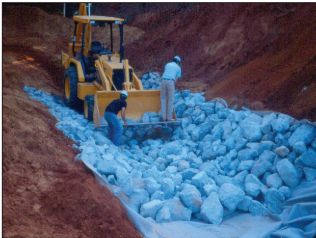
Figure RS-1 Hand Placing Riprap.
