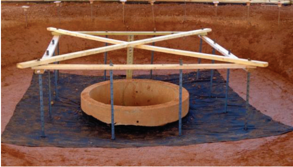
Figure IP-1 Silt Fence Inlet Protection installation showing geotextile underlayment, steel T-posts, 2 x 4 bracing, and dewatering device.
