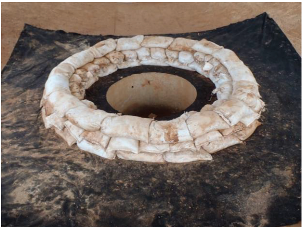
Figure IP-4 IP-5 Sand Bag Inlet Protection installation.
