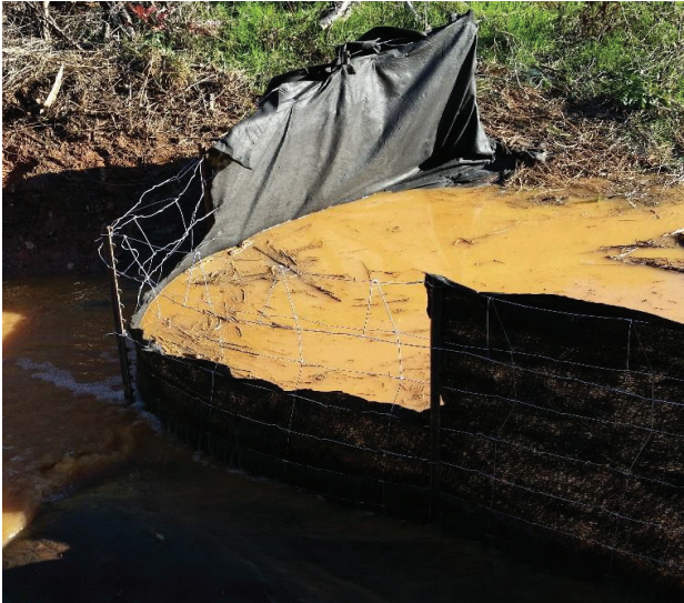
Figure CD-7 Silt Fence Check Dam
