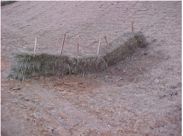
Figure ST-2 Straw Bales Sediment Trap
