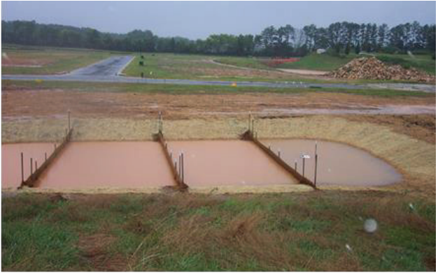
Figure EDS-1 Sediment Basin
