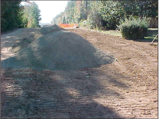
Figure TSG-1 Topsoil to be Spread.
