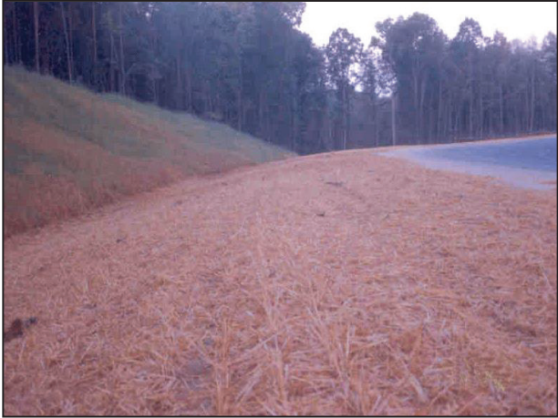
Figure MU-1 Crimped Straw Mulch.
