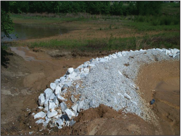
Figure RD-3 Typical Rock Filter Dam
