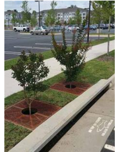
Filterra® Bioretention System by Contech® Engineered Solutions
