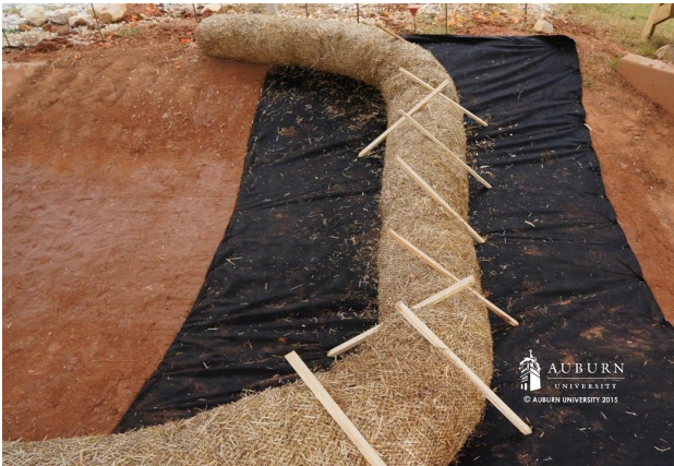
Figure CD-4 Wattle Check Dam
