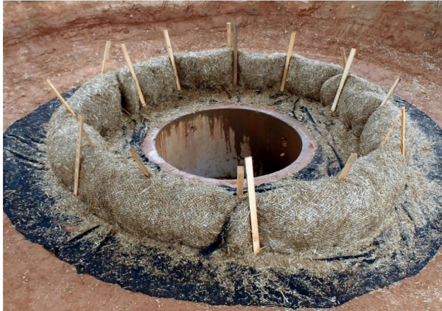
Figure IP-5 Wattle Inlet Protection Installation. (Photo courtesy of AU-SRF. See Appendix for CAD files)
