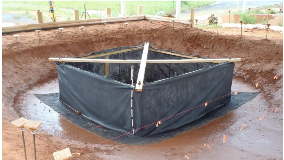
Figure IP-1 Silt Fence Inlet Protection Installation. (Showing silt fence, geotextile underlayment, steel T-posts, 2 x 4 bracing, and dewatering device.) (Photo courtesy of AU-SRF. See Appendix for CAD files)
