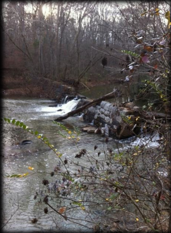
Pre dam removal
