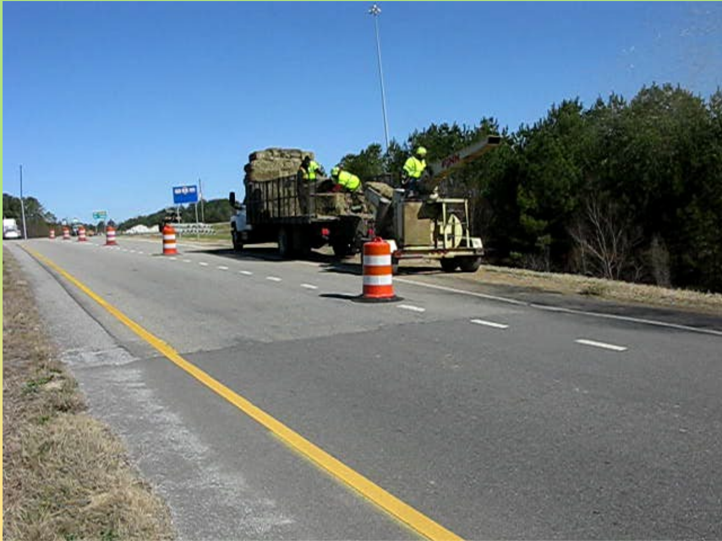
Mulching Crew and Blower:
